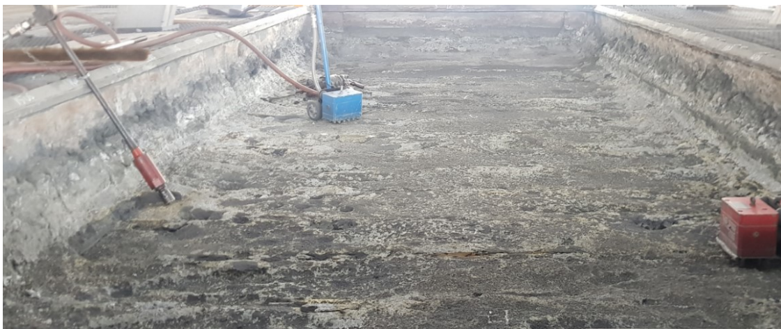
Figure 9. Test II, view of the cathode block surface at the age of 972 days.
