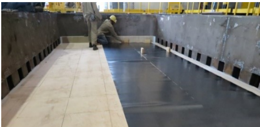
Figure 1. Cell construction using graphite foil.
